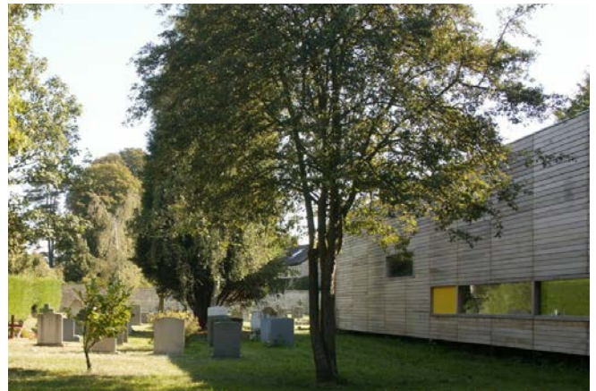
Figure 87: North Building. All Saints Church. © Tim Soar 2018
