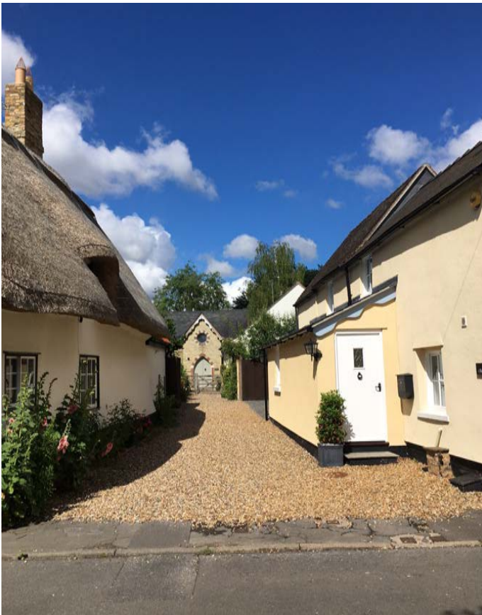
Figure 102: View towards the former Congregational Church with the former bakery on the right hand side
