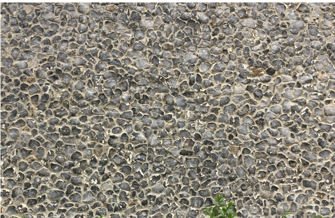
Figure 68: Pebble and knapped flint walls
