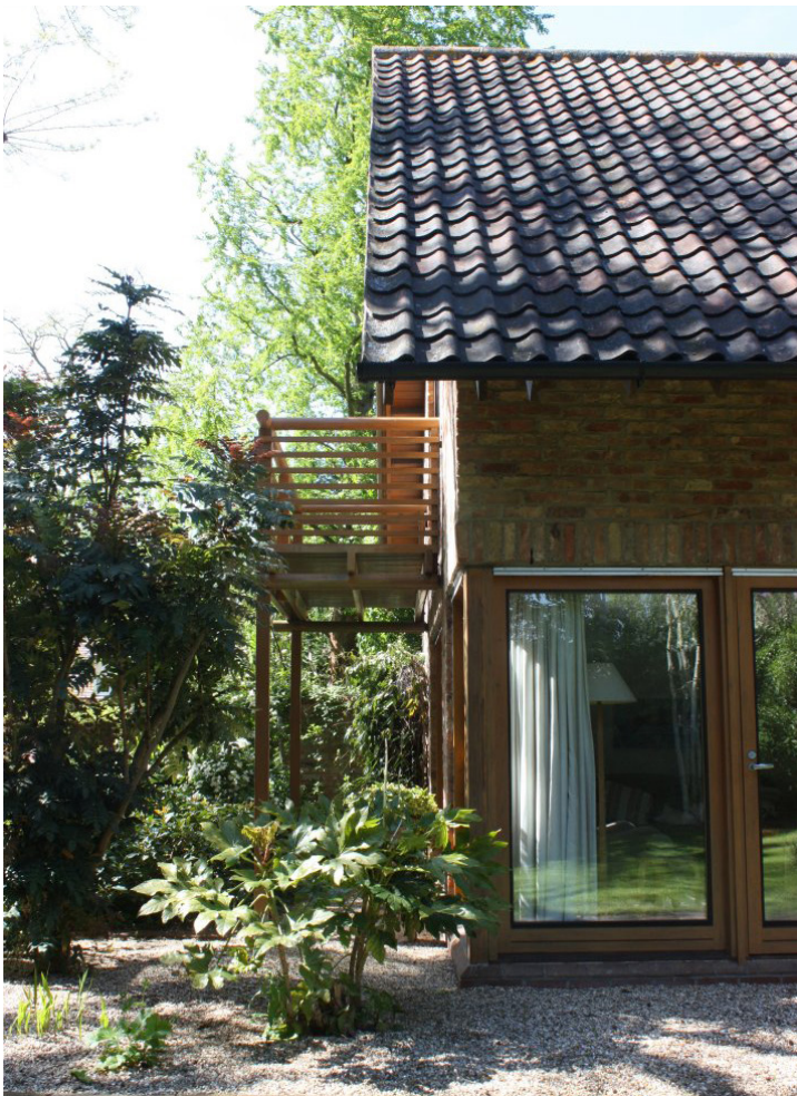
Figure 88: Kings Garden, 29 High Street.
