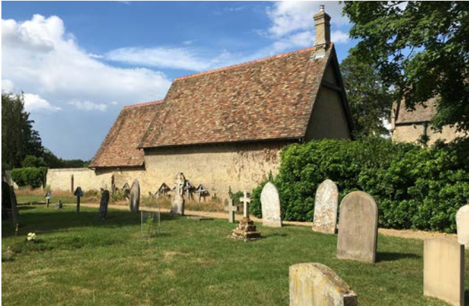
Figure 80: Priesthouse outbuildings, 33 Church Street
