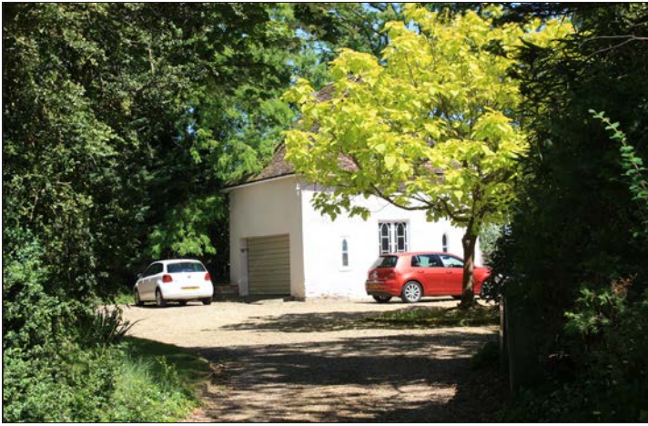
Figure 70: Kings Farmhouse Dovecote, 21 High Street.
