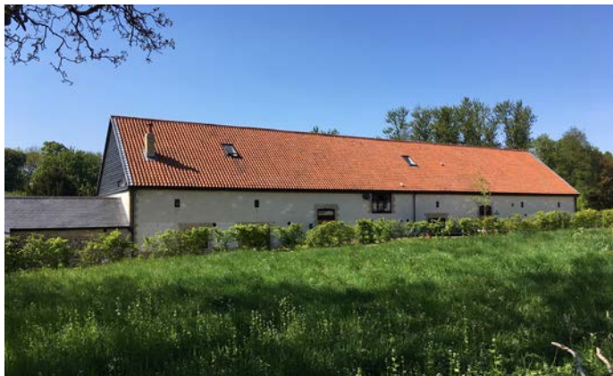
Figure 107: Terraced housing in Great Shelford
