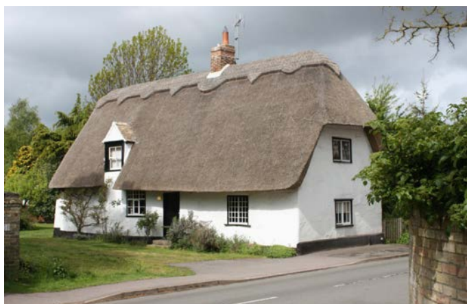
Figure 61: White's Farmhouse. 26 High Street.
