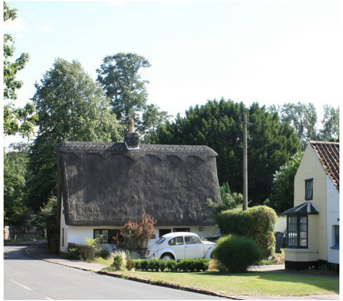
Figure 19: Toll House, 14 Whittlesford Road
