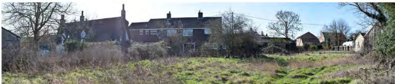
Fig.3.1 Southern view from the site toward Burgess Road demonstrating the built form that exists
