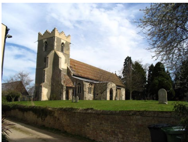
The church viewed from St John's Lane
