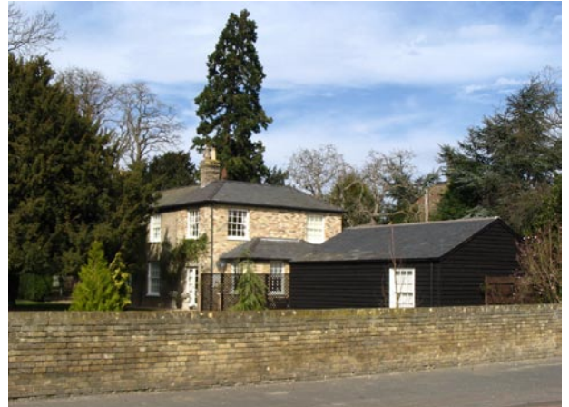
The rear of the Old Rectory
