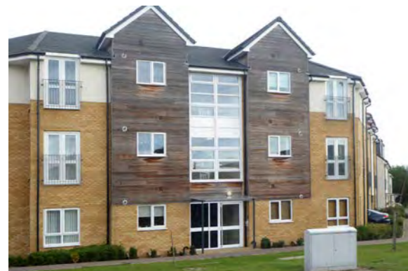
Fig. 82 - Corner blocks with lit stairwell are unsuitably suburban
