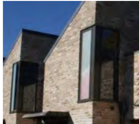
Fig. 68 - Corner windows and terraces are positive features
