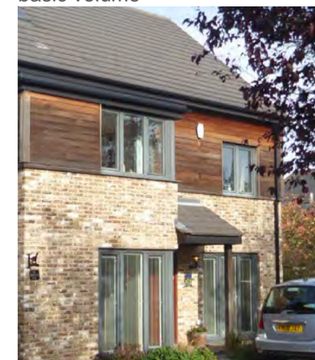
Fig. 58 - New porch and good quality windows
