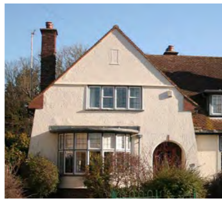
Fig. 67 - Elegant combination of large windows and roof geometry
