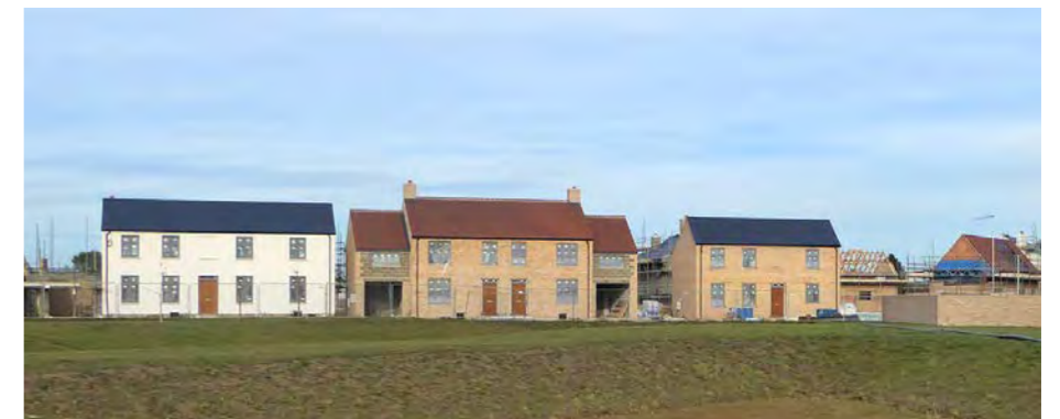
Fig. 89 - Hard and compact frontage onto the countryside creates an unsuitable edge to village development
