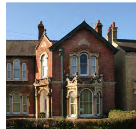
Fig. 4 - Exuberant Victorian building near Saffron Road (B)
