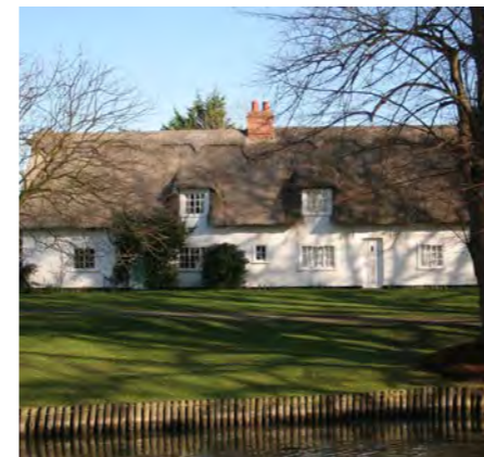
Fig. 3 - Farmhouses now at the core of the village, on the Green (A)
