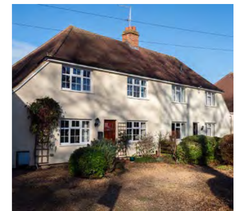
Fig. 5 - Interesting 1920-30 houses along New Road (C)
