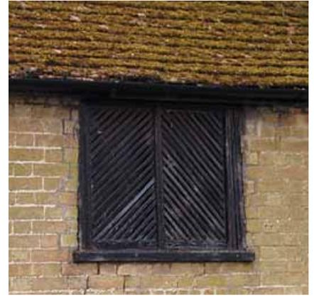
Early windows were usually horizontal in emphasis and typically opened using horizontal sliding sashes (left). Dormers were of 'cat slide' form (centre). Rooms used for storing cheese (right) were ventilated by slatted windows.
