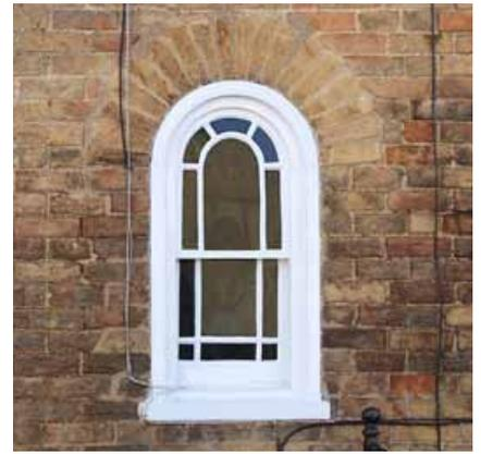
Later windows were of vertical emphasis, either divided into equal lights (left) or decorated with narrow margin lights (centre). Lintels were often of gauged brickwork. Small, round-headed windows (locally known as 'poor windows') are found on a number of houses – usually towards the front of a side wall.
