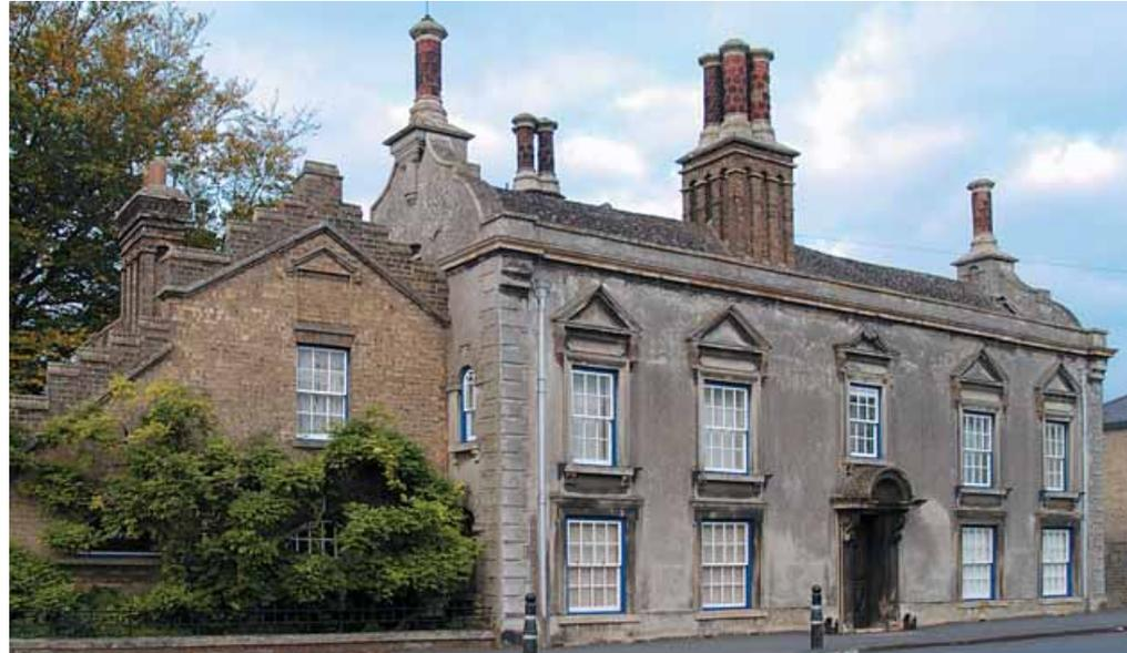
later cased or rebuilt, usually in red brick (or yellow brick later in the 19th century) laid in Flemish bond.
