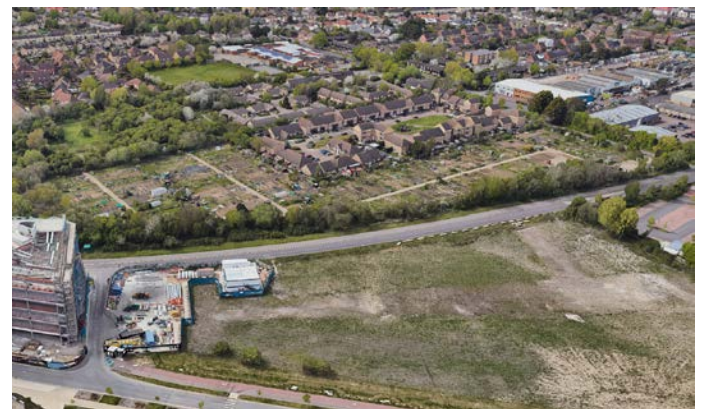
Fig. 106 Existing Western Edge Condition
