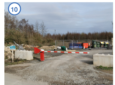
Fig. 59 View towards NE from aggregate works service road
