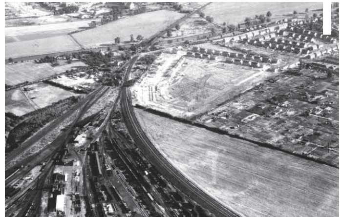
Fig. 46 Aerial view of long welded track plant
