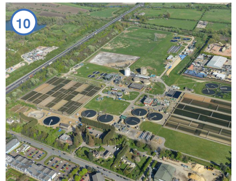
Fig. 40 Waste Water Treatment Plant
