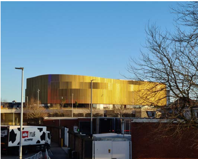
Fig. 3 ACME work: Swansea Arena, Swansea
