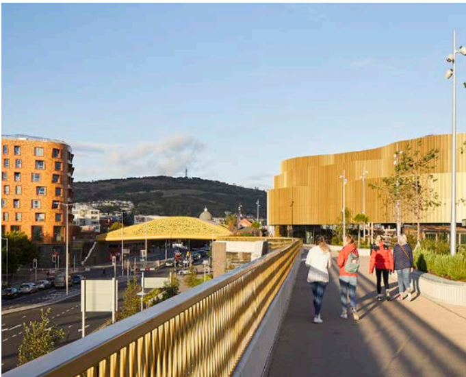
Fig. 8 ACME work: Copr Bay, Swansea
