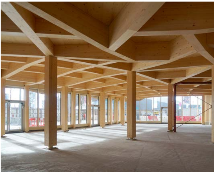
Fig. 7 ACME work: Stratford Pavillion, London
