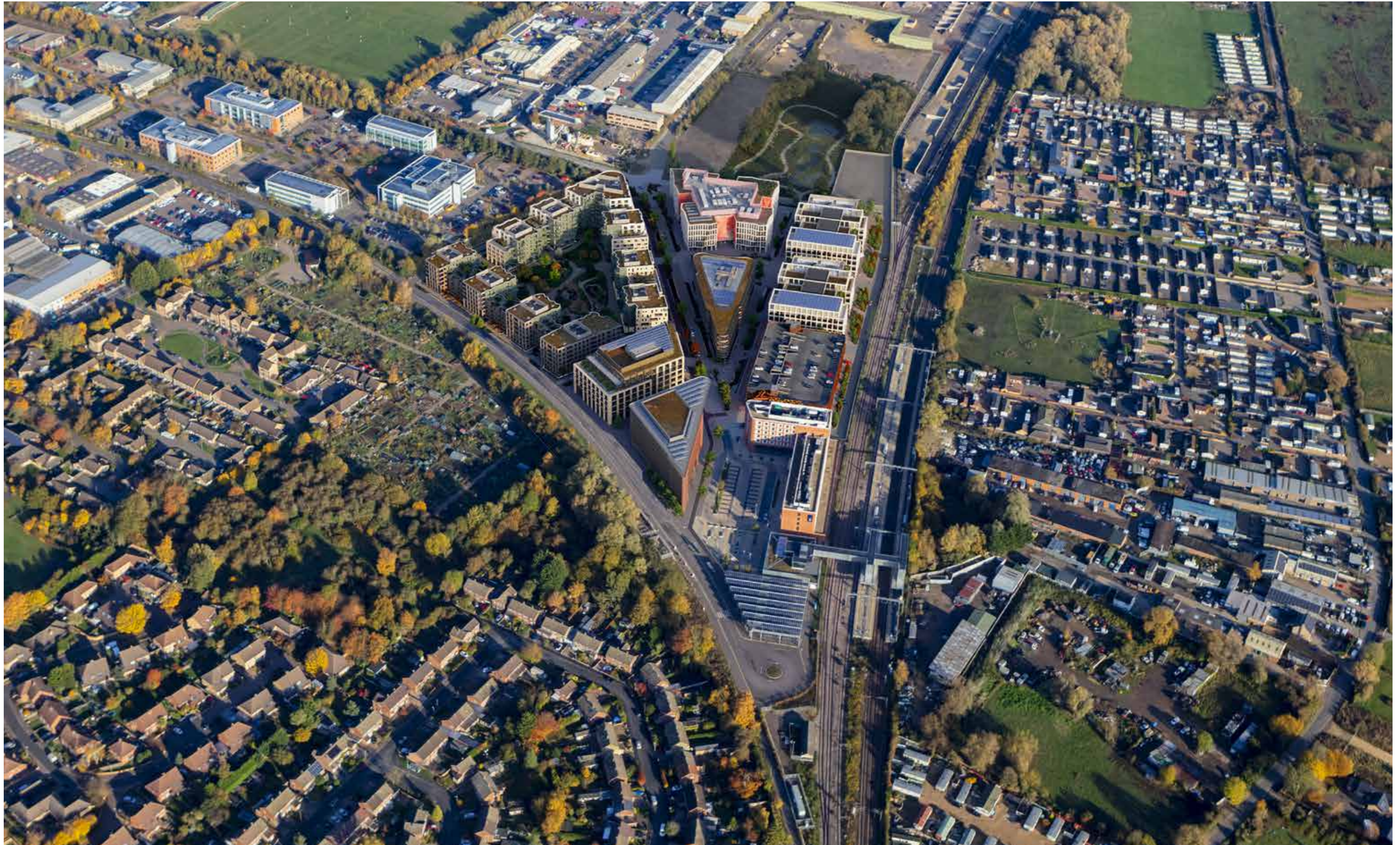
Aerial view looking north
