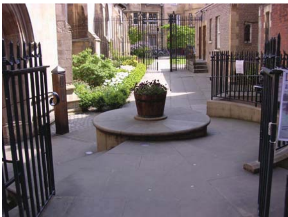
Disabled access ramp and steps introduced into a tight site at the Michaelhouse Centre, Cambridge.
