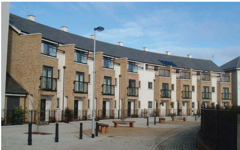
Vertical bays on similar terrace to the one above, creates a primarily vertical emphasis, giving the impression of a shorter and taller terrace than the one above.
