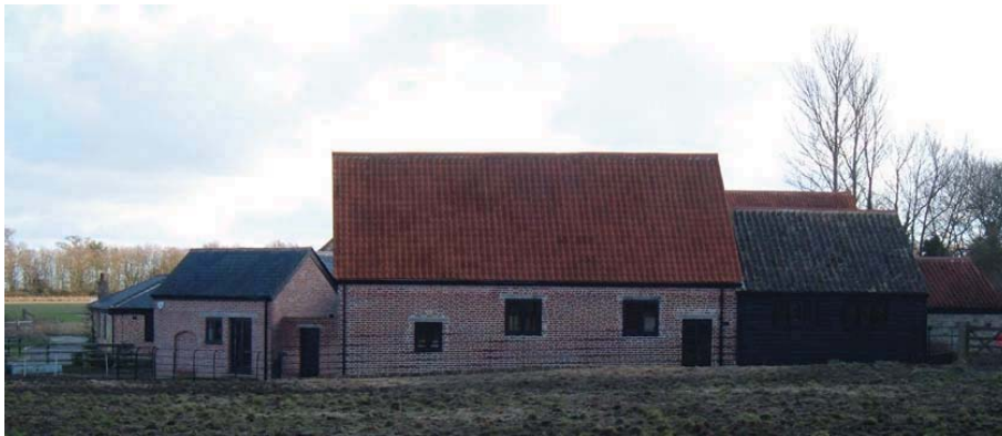
Kings Road, Hardwick, view from the main road.
