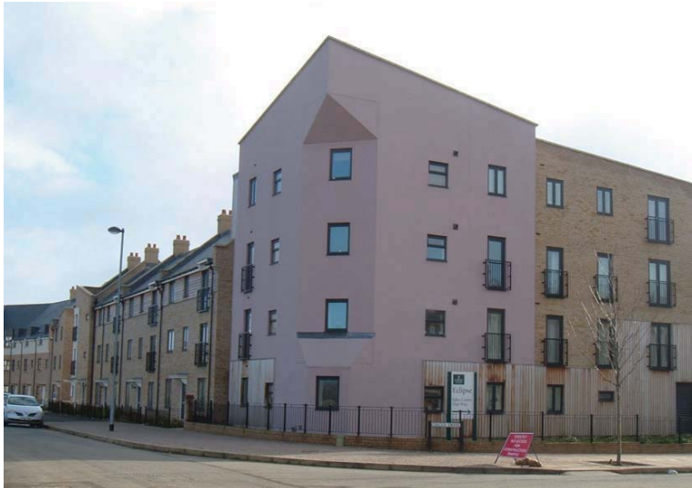
A feature corner building acting as a way marker, Orchard Park.
