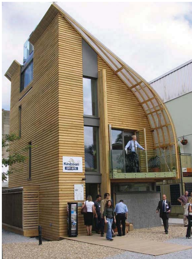
The asymmetrical Kingspan building at the Off-Site exhibition, BRE Watford.
