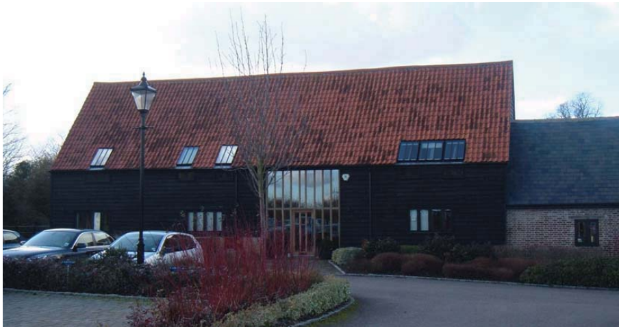
Kings Road, Hardwick, view of the main barn from the car park.
