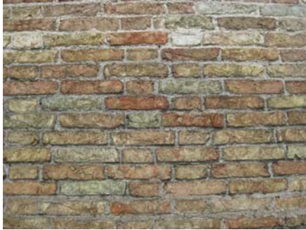
(left) Early gault brick in garden wall bond (right) Red brick in Flemish bond
