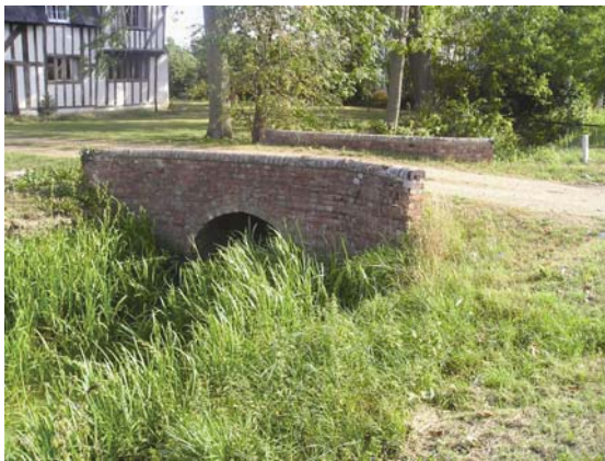
(left) Simple brick bridge
