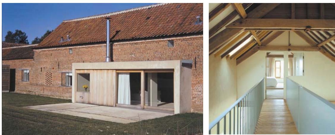
A contemporary addition and interior to a converted barn. ('Quaker Barns', Hudson Architects)
