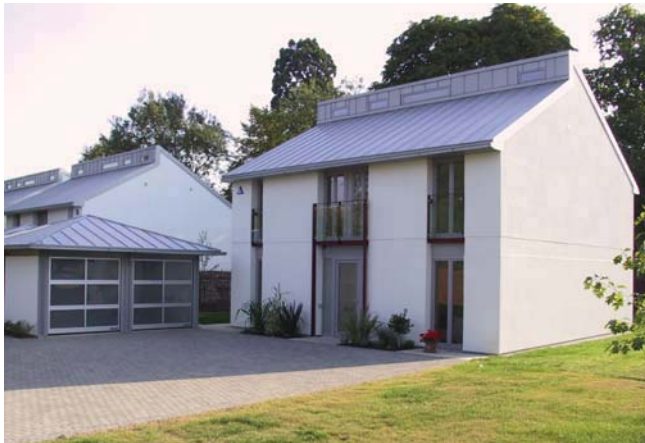
Infill houses, Melbourn. The rendered walls and tall window proportions make reference to the listed house, with contemporary metal roofing and window frames (Plum Developments).
