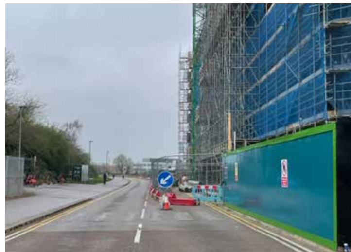
⑧ View along Cambridgeshire Guided Busway
