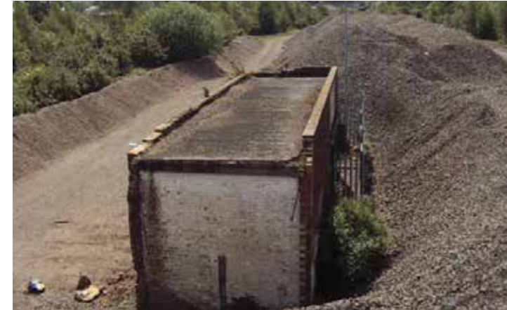
2012 - Remaining building - sub station
