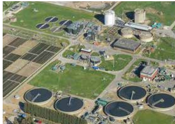
④ Waste water treatment plant
