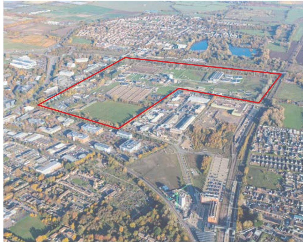
Waste treatment plant site
