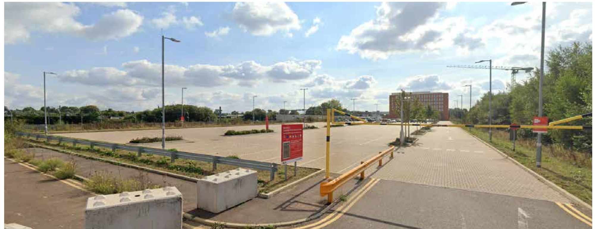
View of carpark looking north
