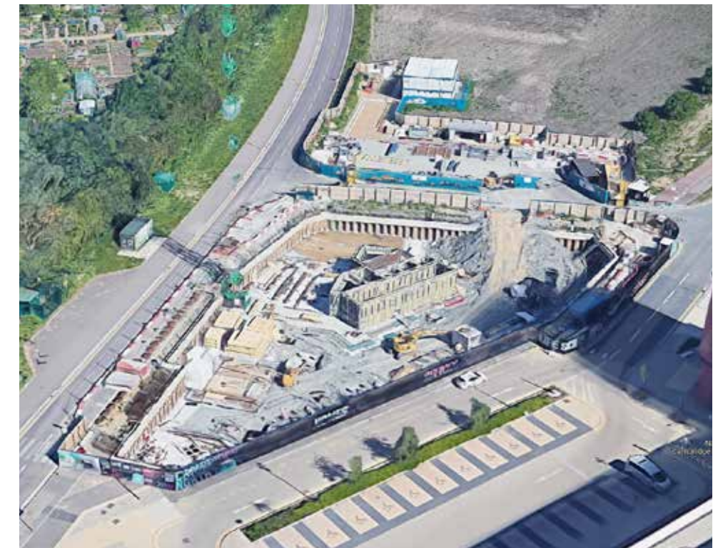
Site currently under construction
