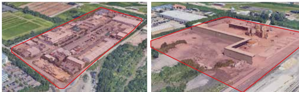
2 AGGREGATE WORKS & INDUSTRIAL ESTATE High volume of heavy vehicles and traffic along roads servicing the estate
