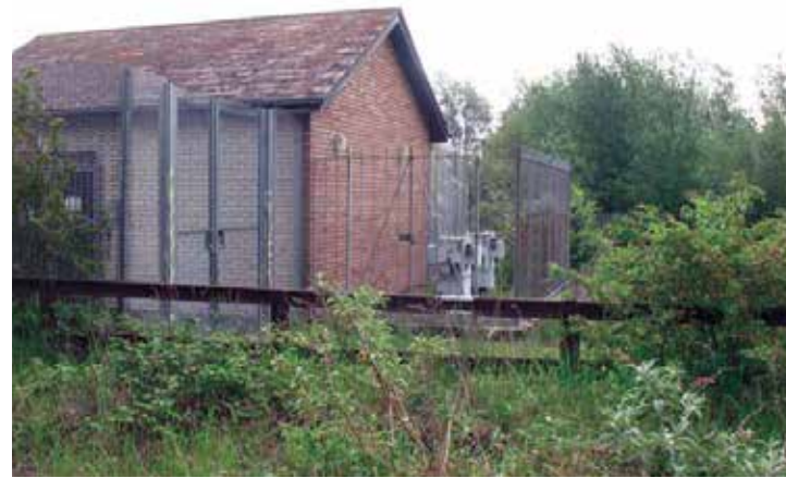
2012 - Remaining building - generator building
