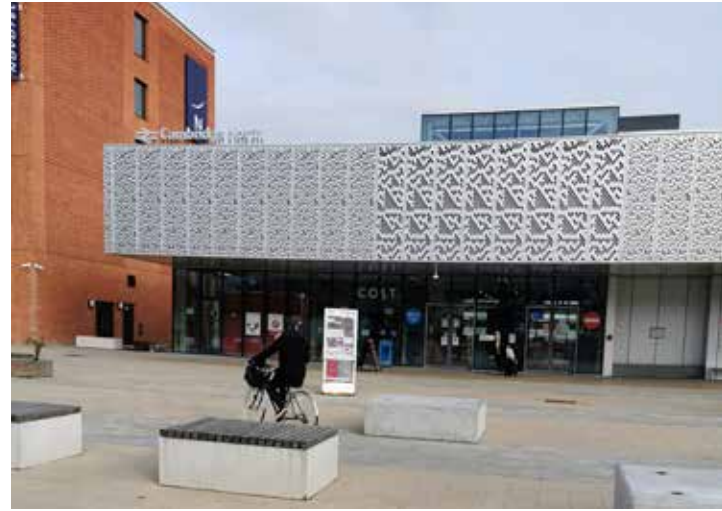
① Cambridge North Station
