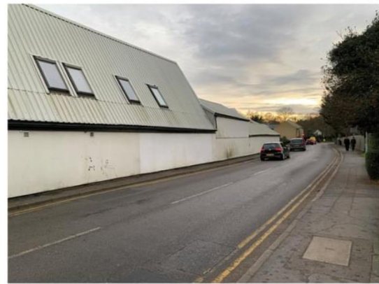
The existing building on site
