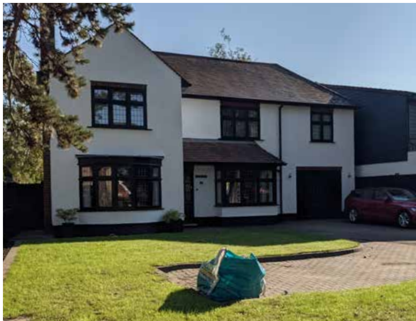
15 Tunwells Lane - 20th Century detached dwelling, modernised
