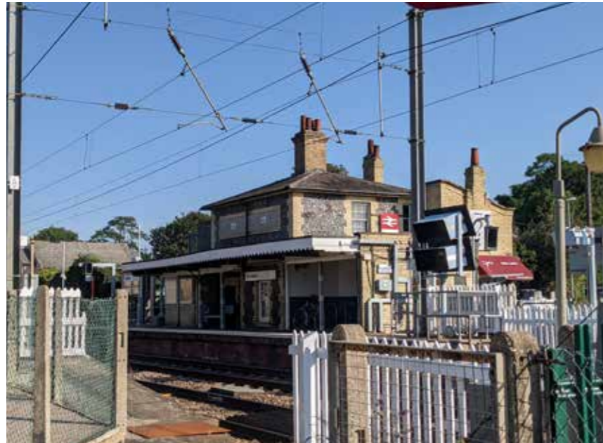
A - To the north of the site is Shelford Railway Station, erected circa. 1845. This building is traditional in design, using a mixture of bricks, a shallow hipped roof and retains many of its original features.
