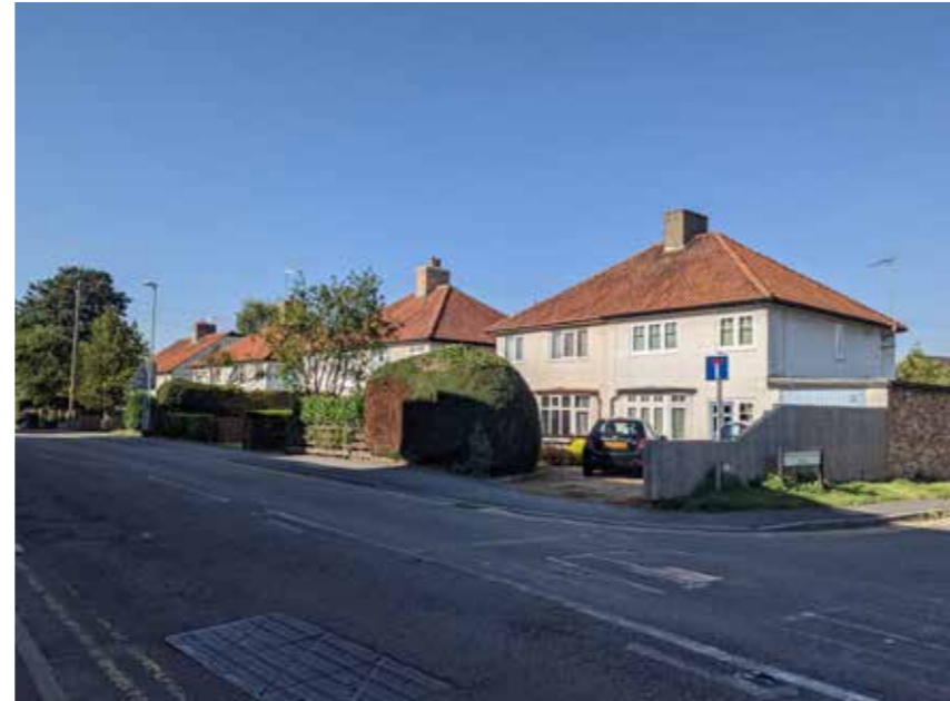
B - To the west of the site, are four pairs of semi-detached dwellings, built in the 1950s.
