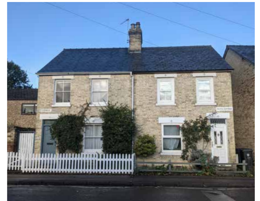
Simple Façades feature on No 1 London Road (Reed House - Top) and Faith and Hope Cottages (Bottom)
