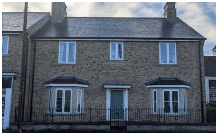
Old School Court - Fronting Woollards Lane
