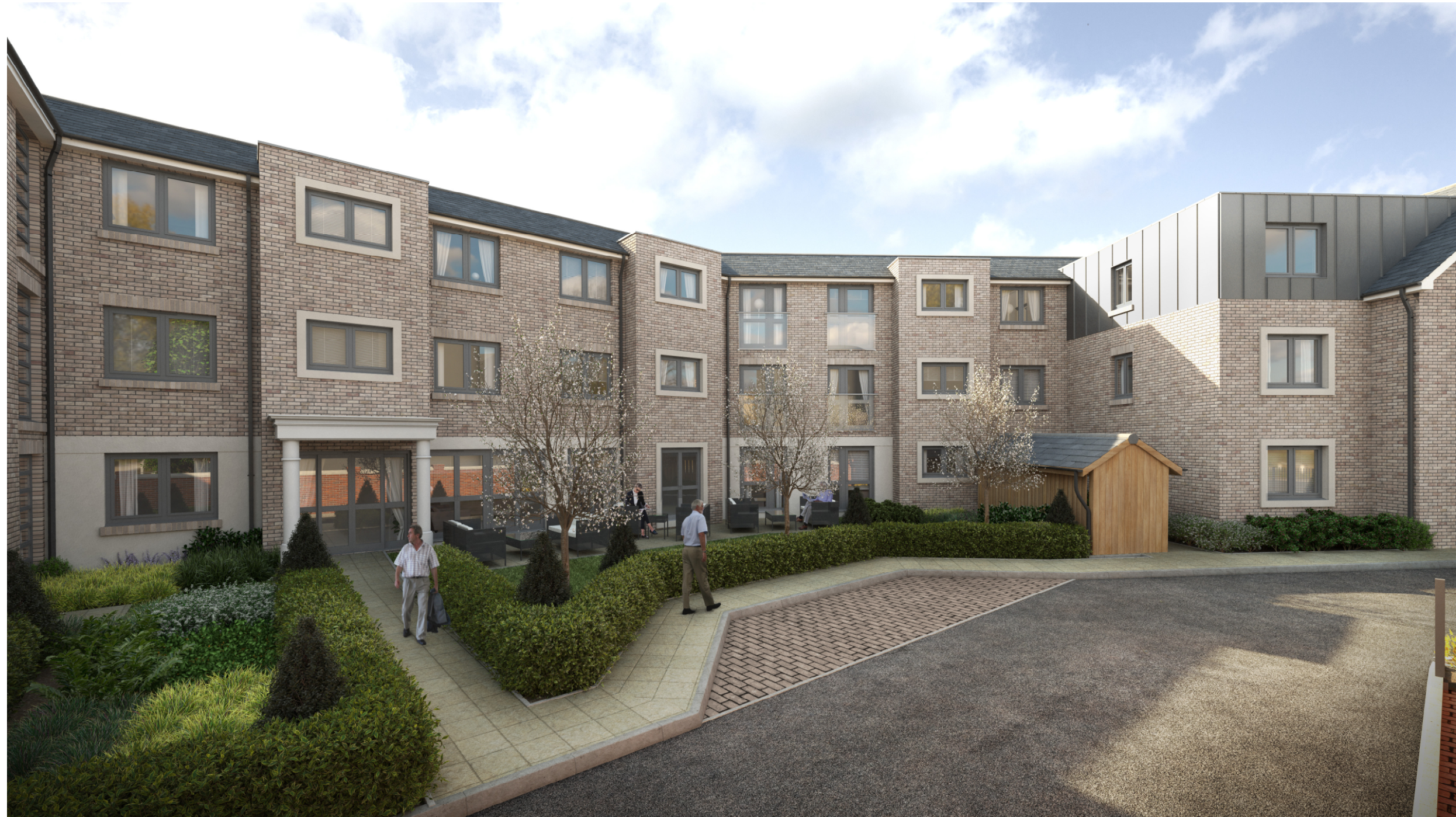
Additional CGI image showing the entrance to the building on the North Elevation
