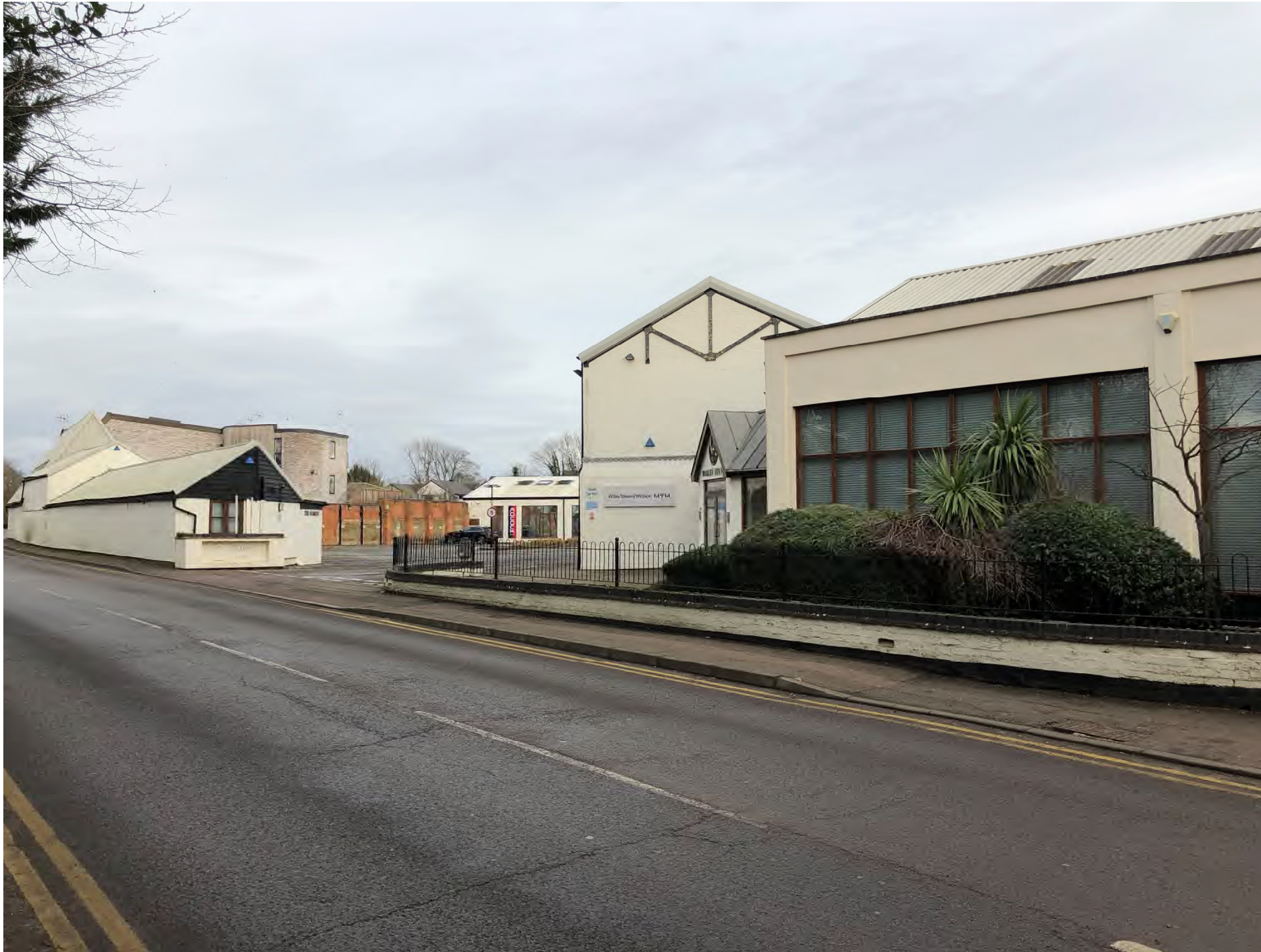
View towards site from Station Road (Pre Demolition of Neighbouring Site)
