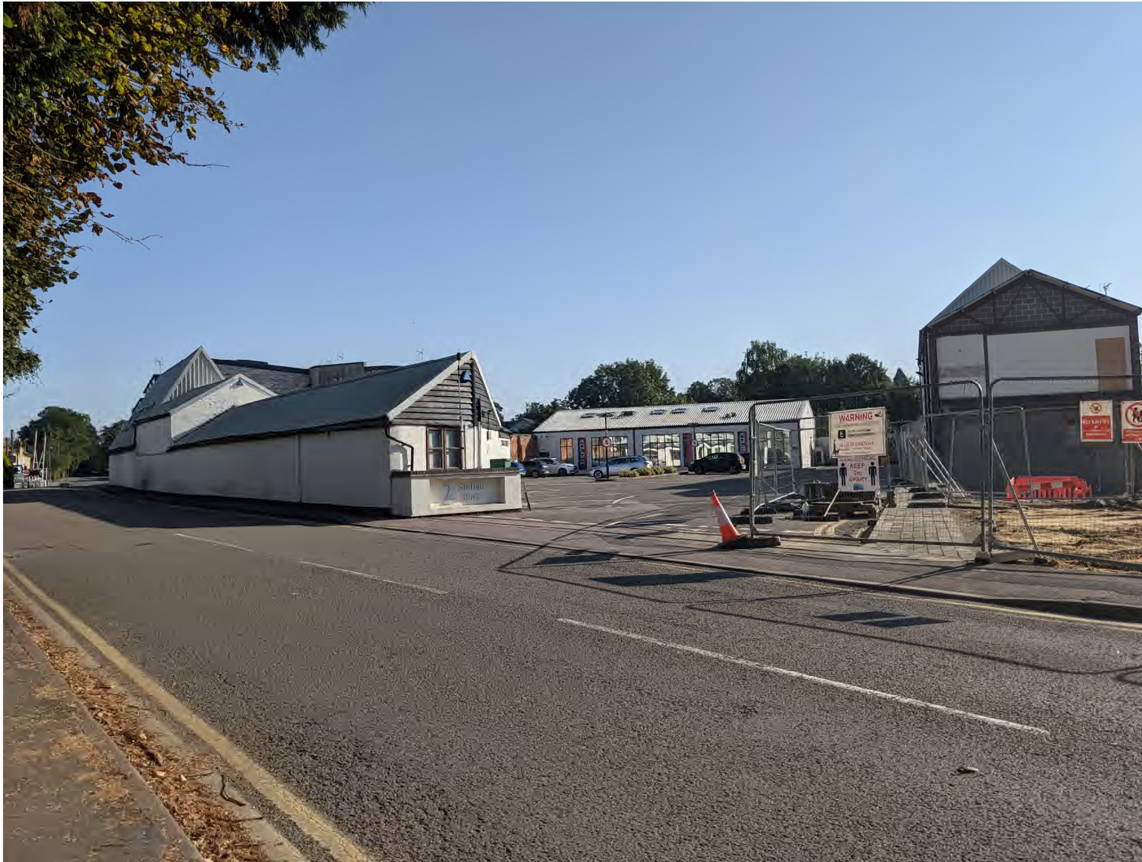
View towards site from Station Road (Post Demolition of Neighbouring Site)
