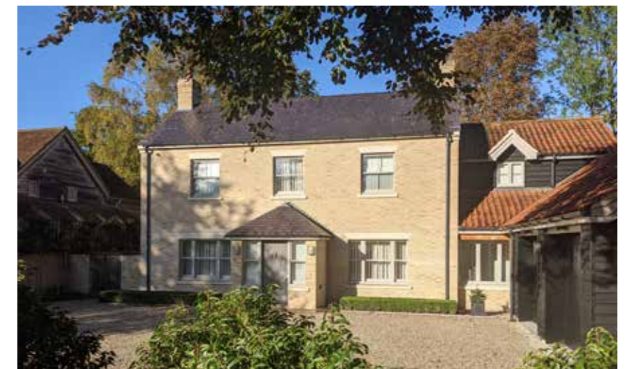
Dandys - Kings Mill Lane - New Build
