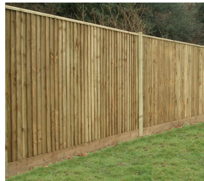
Fence Type 1A: Close Boarded Fence
