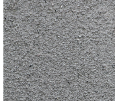
F4. Concrete Paving
