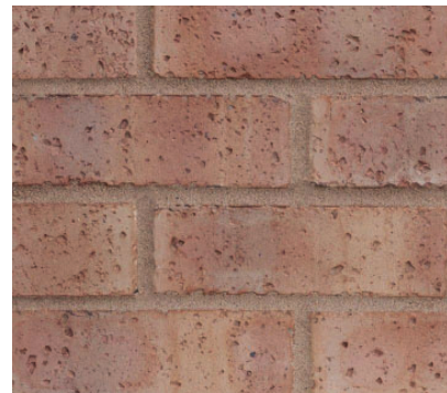
Feature Brick Wall
