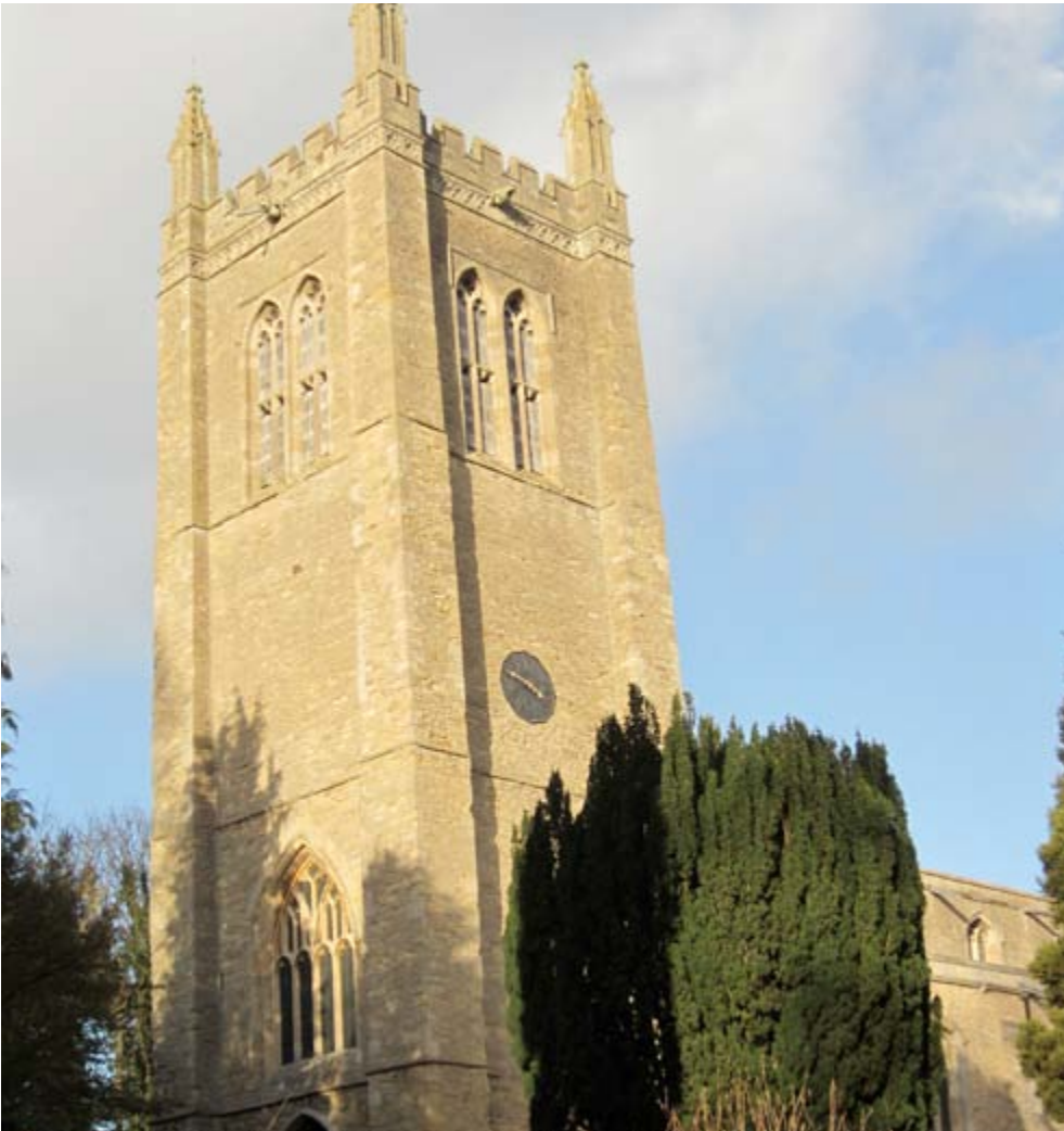
Locally quarried limestone is used in village buildings like this church in Odell.
