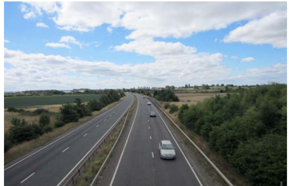
New road infrastructure includes this new section of the A421 linking Junction 13 of the M1 to the A1.
