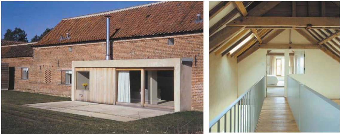
A contemporary addition and interior to a converted barn. ('Quaker Barns', Hudson Architects)
