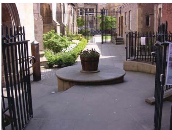
Disabled access ramp and steps introduced into a tight site at the Michaelhouse Centre, Cambridge.
