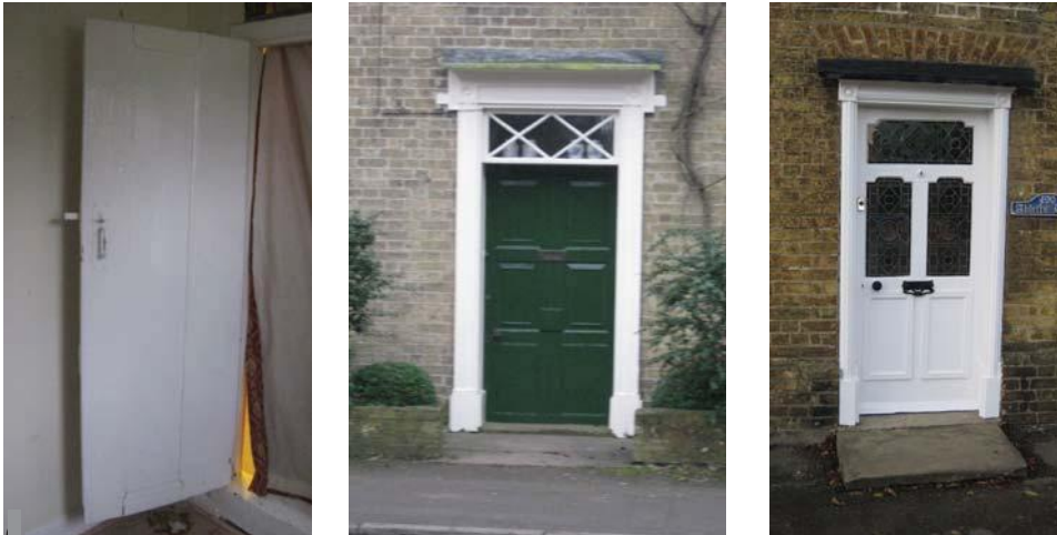
(left) An internal boarded (planked) door (middle) Late eighteenth century door (right) Nineteenth century door
