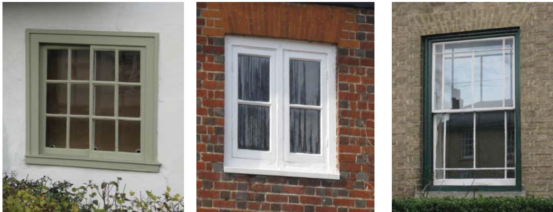
(left) Horizontal sliding (Yorkshire) sash window (middle) Side opening casement window (right) Vertical sliding sash window (with circa 1800 marginal light design)
