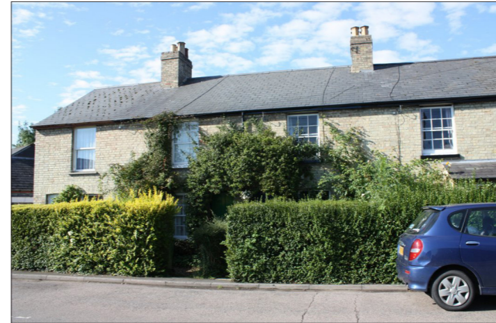
Figure 67: Terrace, 21-27 Hauxton Road.
