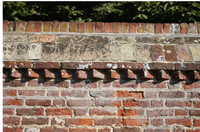
Figure 77: Boundary wall. The Manor House, Bridge Lane.
