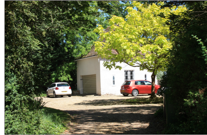
Figure 70: Kings Farmhouse Dovecote, 21 High Street.
