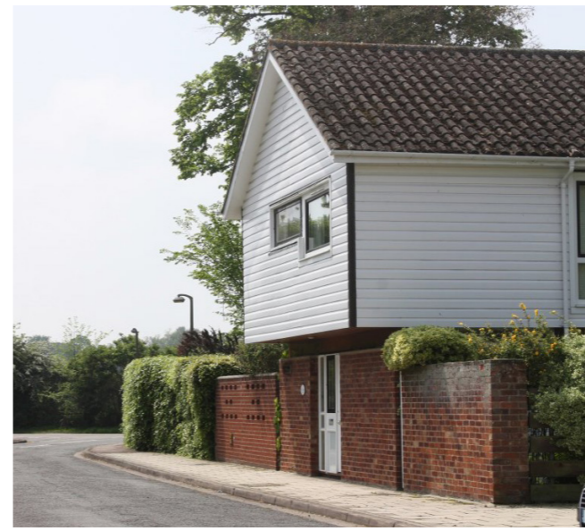
Figure 18: 1 Courtyards, Whittlesford Road
