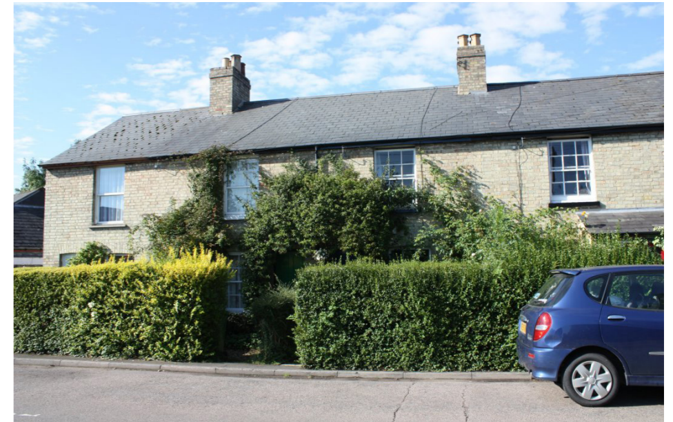
Figure 51: Victorian Terrace, 21-27 Hauxton Road
