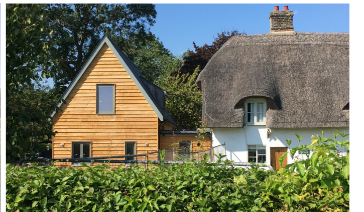
Figure 111: Extension to a listed cottage in Haslingfield
