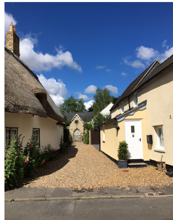
Figure 102: View towards the former Congregational Church with the former bakery on the right hand side
