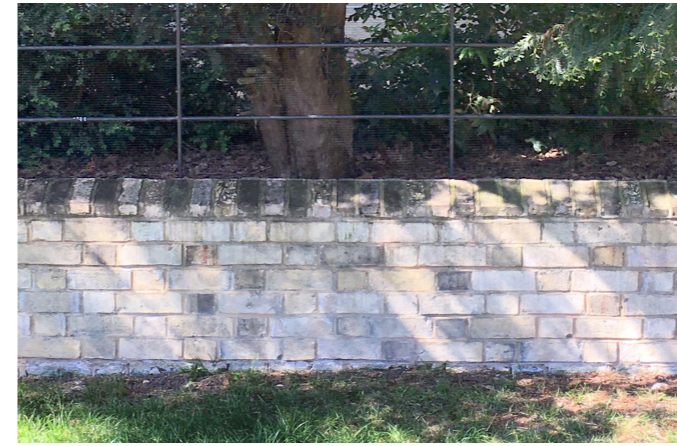
Figure 79: Kirby Lodge, 32 High Street
