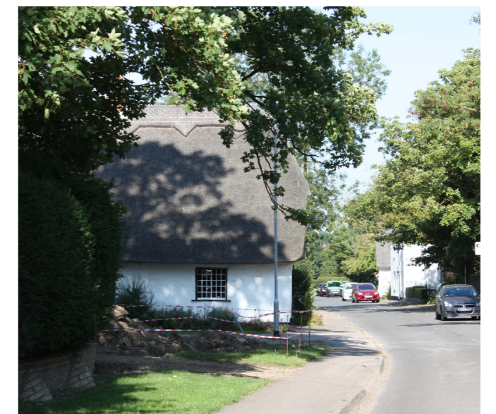
Figure 26: White's Farm House, 26 High Street
