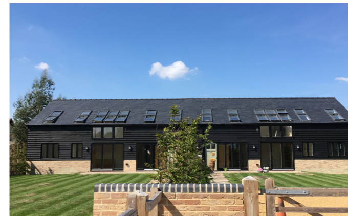
Figure 106: Terraced housing in Haslingfield
