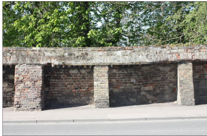
Figure 75: Boundary wall. The Manor House, Bridge Lane.
