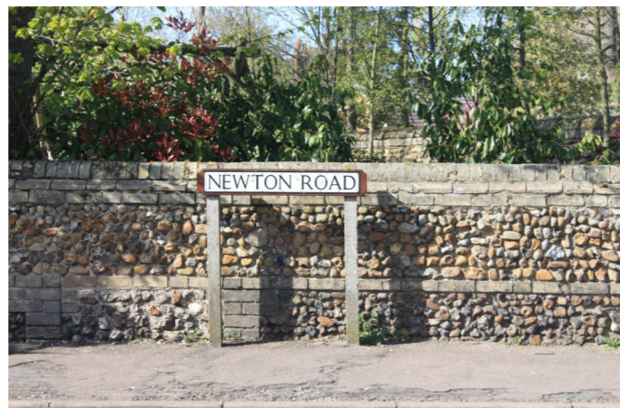
Figure 78: Number 2 boundary wall
