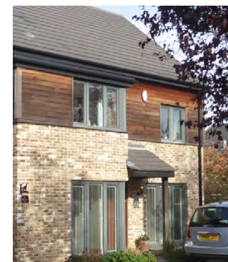
Fig. 58 - New porch and good quality windows
