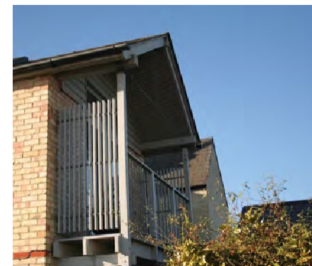
Fig. 55 - Balcony extension adding interest to a plain building
