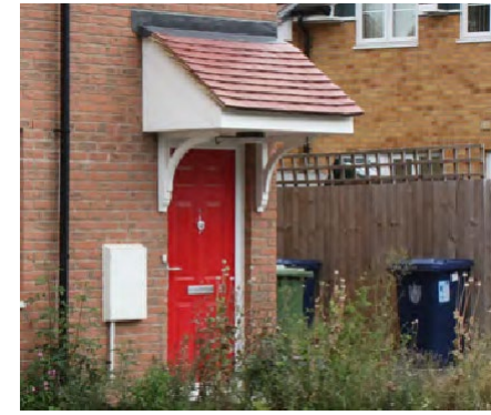
Fig. 88 - Prominent electric box and heavy porch detail can spoil a facade
