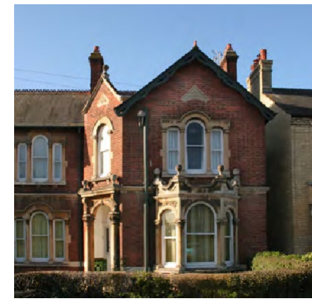
Fig. 4 - Exuberant Victorian building near Saffron Road (B)
