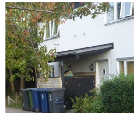
Fig. 89 - Lack of bicycle storage leading to conversion of the bin store
