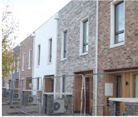
Fig. 80 - Long terraces, which have an inappropriate urban feel
