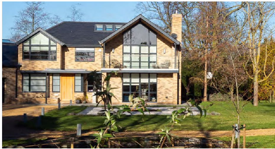
Fig. 65 - Recent house set in the landscape with large windows, balconies and attractive roof articulation
