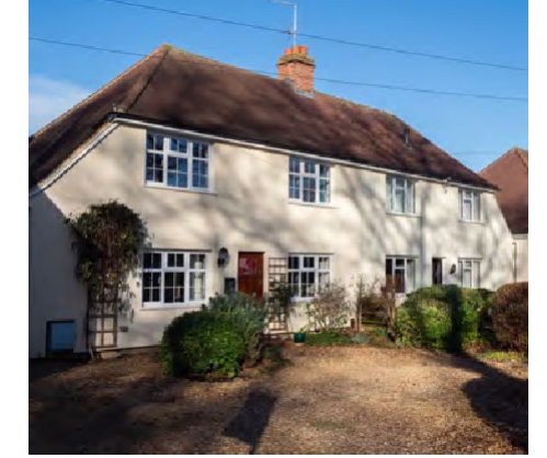
Fig. 5 - Interesting 1920-30 houses along New Road (C)
