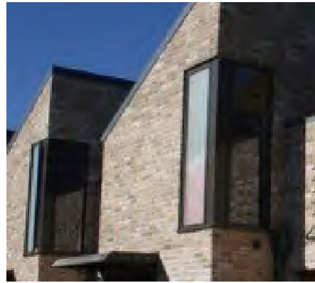
Fig. 68 - Corner windows and terraces are positive features
